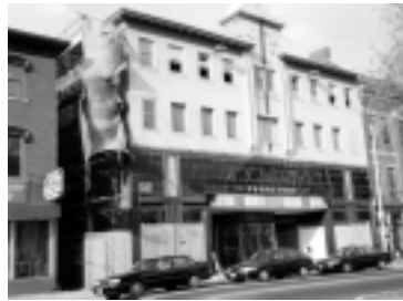
The Armory Revival Company's restoration of the Lilly Building, a mixed-use project that will provide street-level commercial space and residential lofts.
